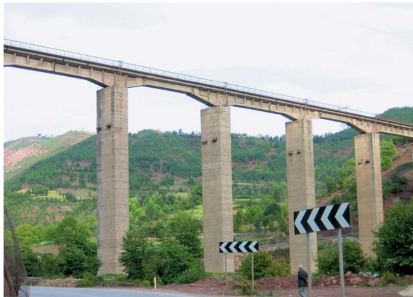
Picture 6 - Viaduct towards Lin
