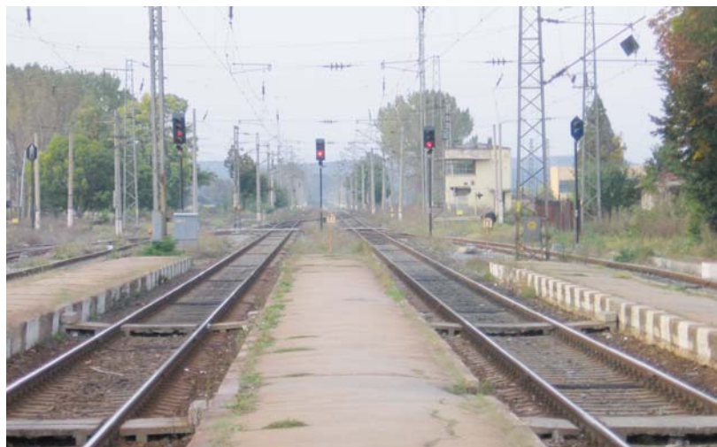
Picture13 - Radomir station: railroad junction between Corridor IV and Corridor VIII
